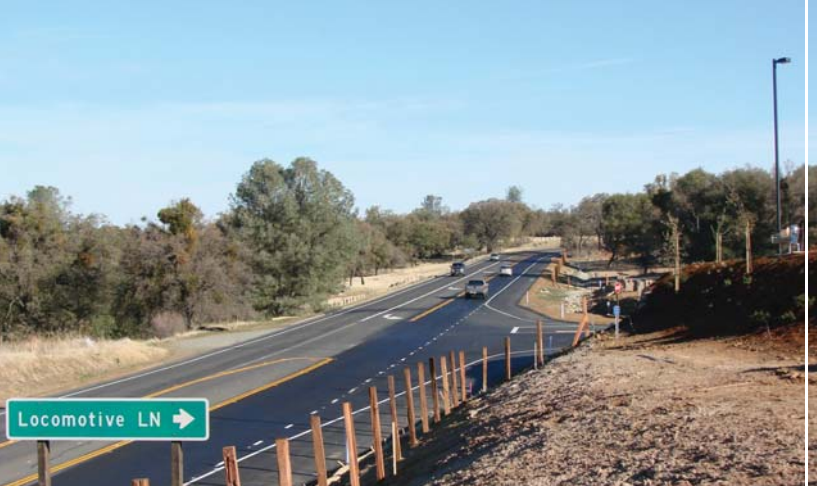
Progress during construction (updated frequently)
