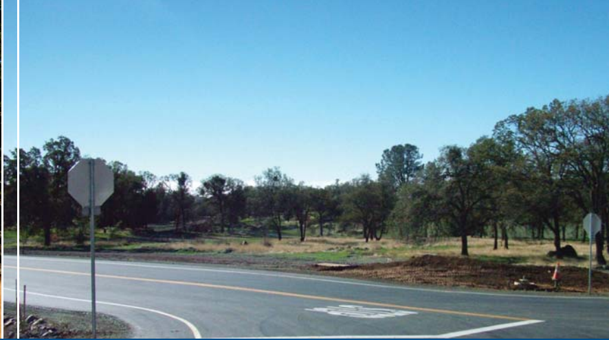
Road construction completed.
