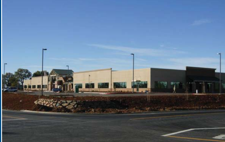
Amador Co. Health Services Building (±50,000 SF)
