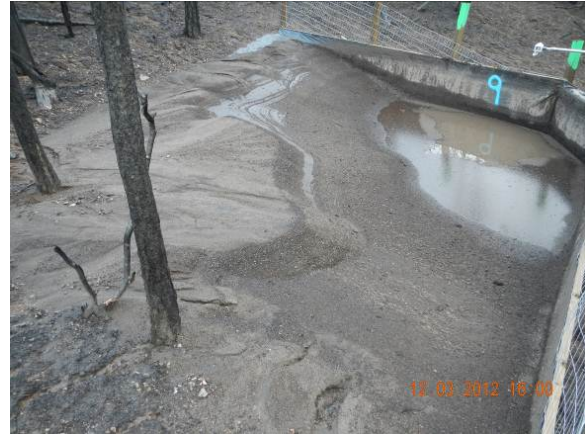
Figure 26. This photograph shows the sediment fence of a control site (site 9), where no salvage logging or contour subsoiling was performed.
