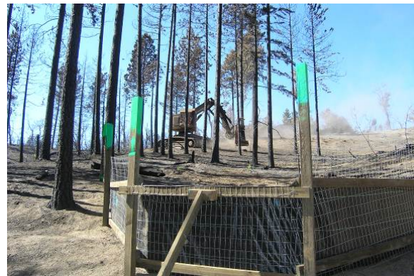
Figure 9. This photograph shows salvage logging plus biomass removal operations occurring upslope of sediment fence.
