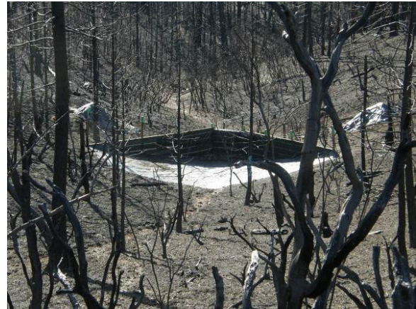
Figure 18. Following the clean-out, the extracted sediment was covered with fabric to protect it from rain.
