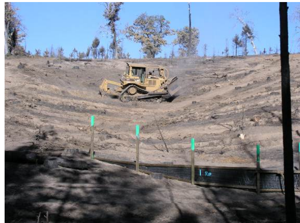
Figure 10. This photograph shows subsoiling done on the contour following salvage logging plus biomass removal.
