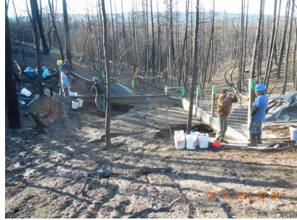
Figure 17. Cleanout crew removing material trapped behind fence and placing into buckets for weighing.
